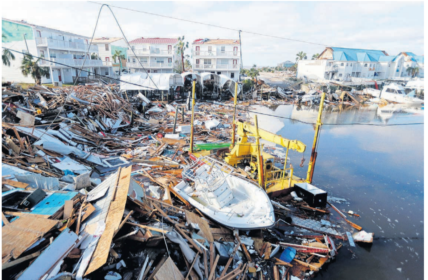
A boat sits amidst debris in the aftermath of Hurricane Michael in Mexico Beach, Fla. Oct. 11, 2018.
